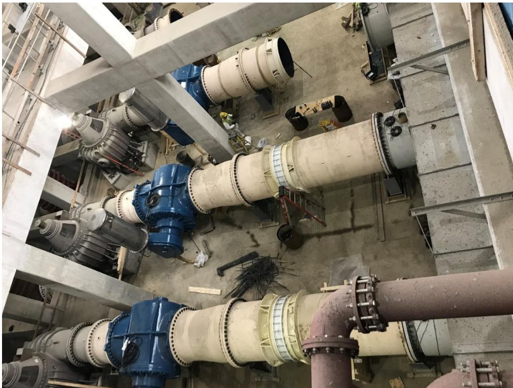
Back River WWTP Headworks IPS Discharge Piping – Jan 2020
